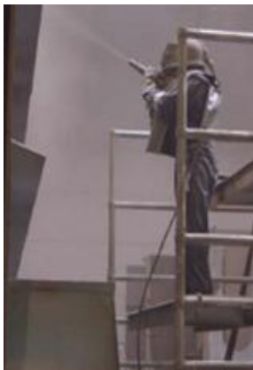
Blasting of the ship section in progress.
